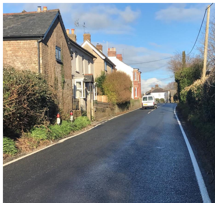
Existing view of North Street (looking north)
