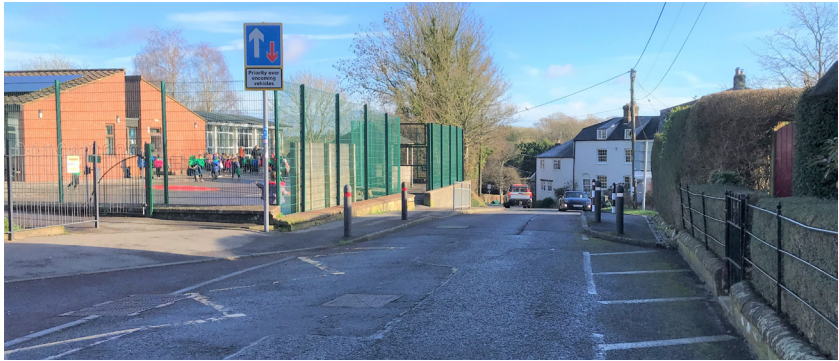
Existing view of West Hill school frontage (looking east)
